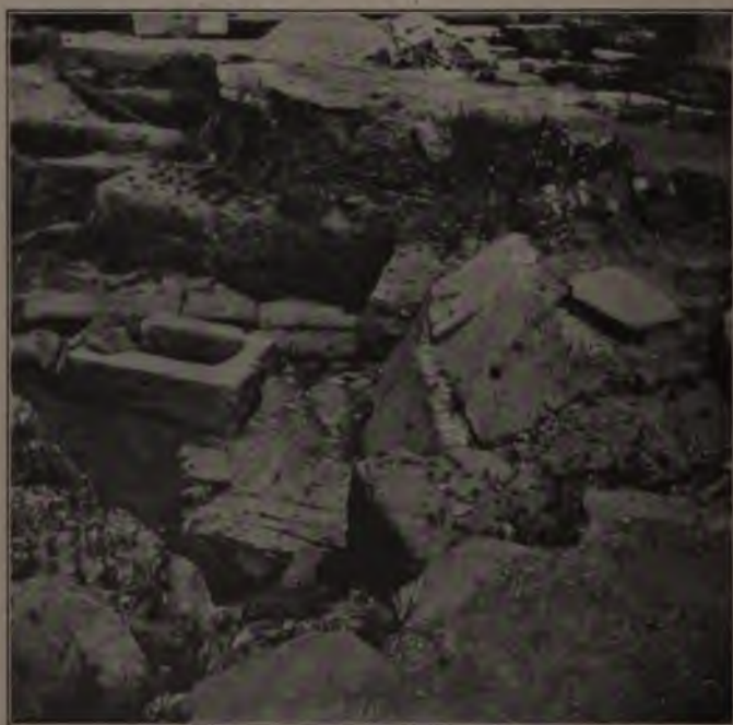
FIG. 50.—SHALLOW PIT, AND VAULT OF THE CLOACA MAXIMA.
